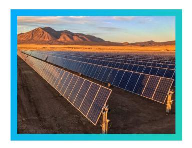
ENGIE developed and installed a 3 MW single-axis tracking solar array in Carrizozo, New Mexico for Otero County Electric Cooperative. ENGIE now operates the project.
